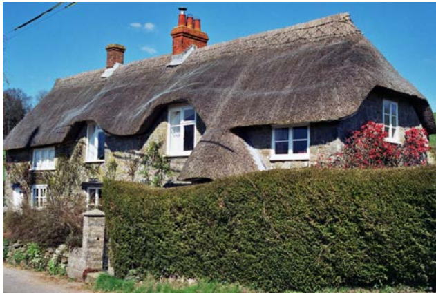
An Old Style Thatched Cottage. Note the Wooden Casement Windows, the Thatched Porch, Brick Chimney Stacks and Stout Hedge. Straw for thatching has been grown and harvested in the village for some time, and is a very acceptable if expensive material
