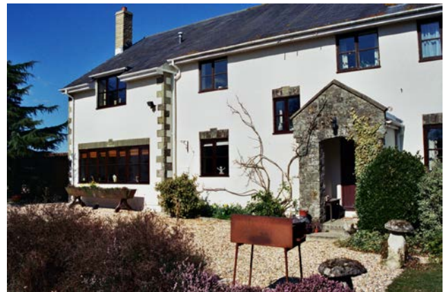
A Modern House with Rendered Walls, Stone Quoins and Porch, and Stained Windows. More modern in appearance than the previous houses, this is nevertheless a very pleasing building
